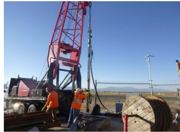
Inserting pump for over-pumping
