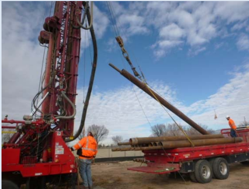
ARCH rig raising drive casing and drill string
