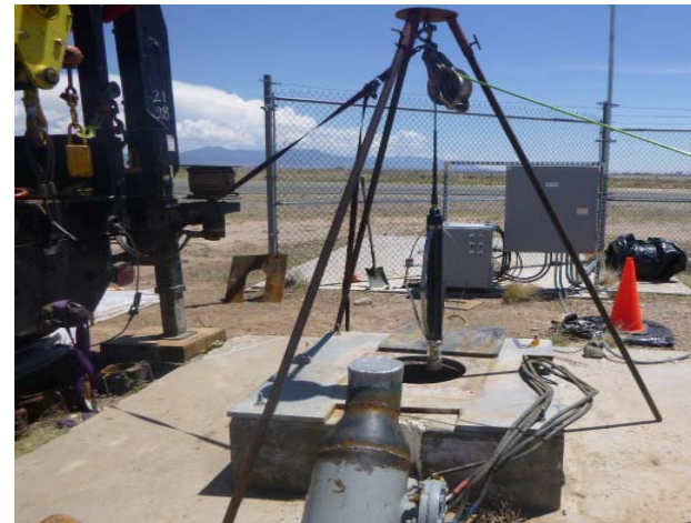
Lowering video camera into well
