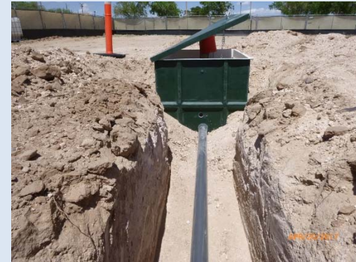
Double-walled conveyance piping being laid to vault
