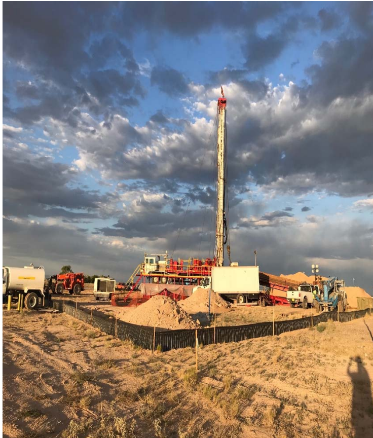
Drilling Rig used for KAFB-106IN2
