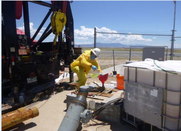
Injection well KAFB-7
