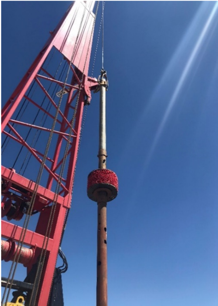
Brush/swab assembly for cleaning
