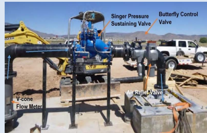
Installing above-grade valves, meters, and piping at injection well KAFB-7
