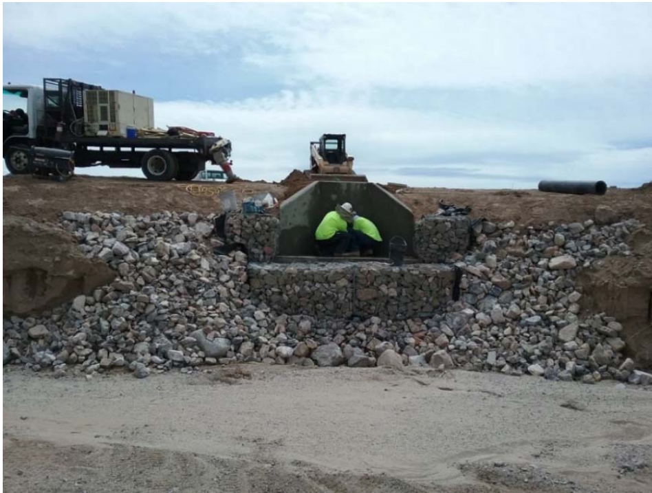
Field crew working on construction of the NPDES outfall
